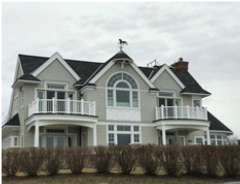
Recently constructed new Victorian style summer cottage on Jerusalem Road
