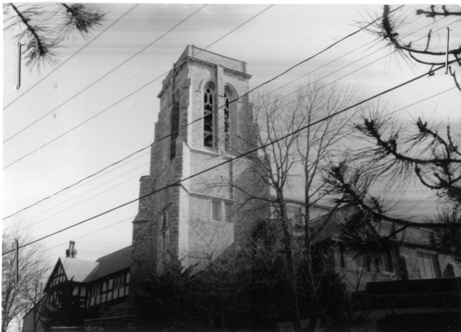
Extreme southeast end of District. St. Stephen's Church, Highland Avenue.
